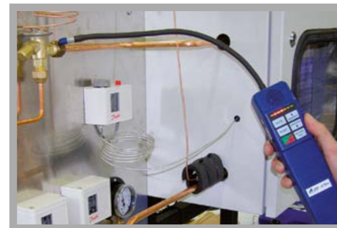
Leak test at the expansion valve of the fully assembled system
