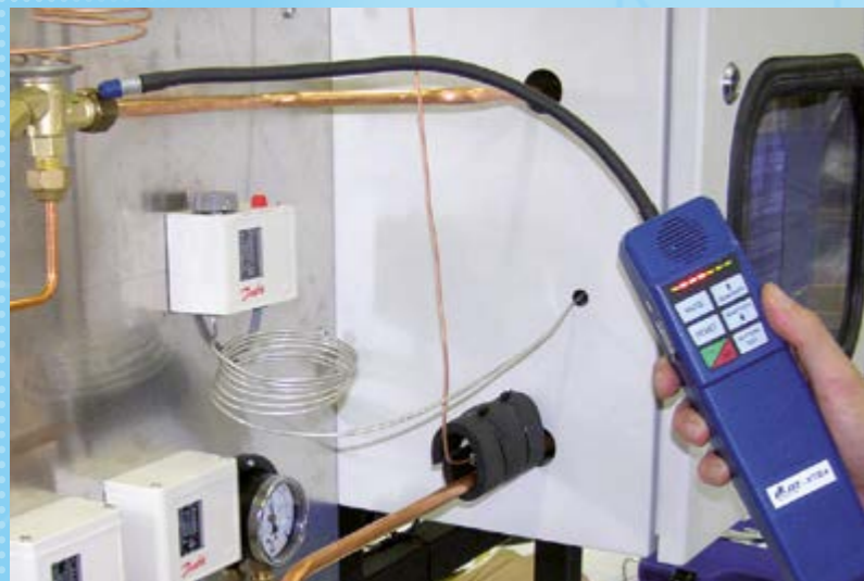
Leak testing at expansion valve
