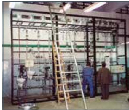
Installation of system at customer's site
