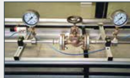
A corresponding measurement station has been incorporated into the measuring section to record a valve characteristic.
