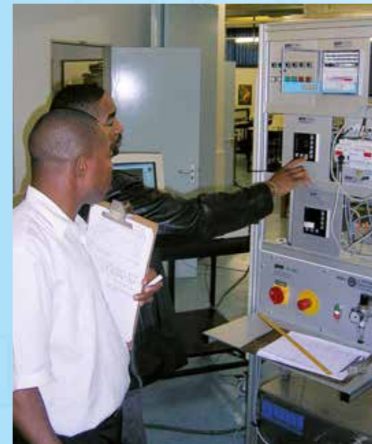
Setting on a digital controller
