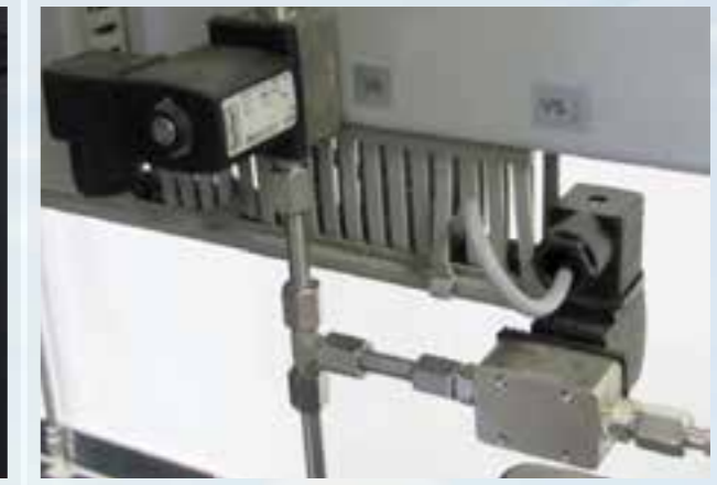
Solenoid valves in heating water circuit
