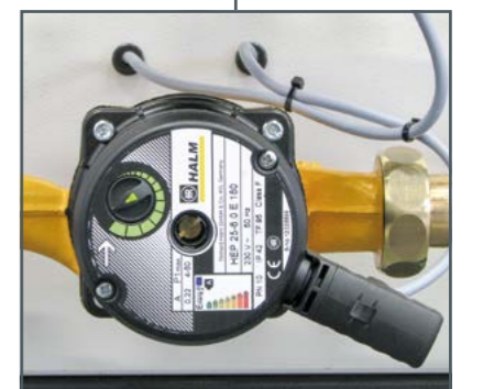
Energy-efficient circulation pump with adjustable differential pressure control (efficiency class A)
