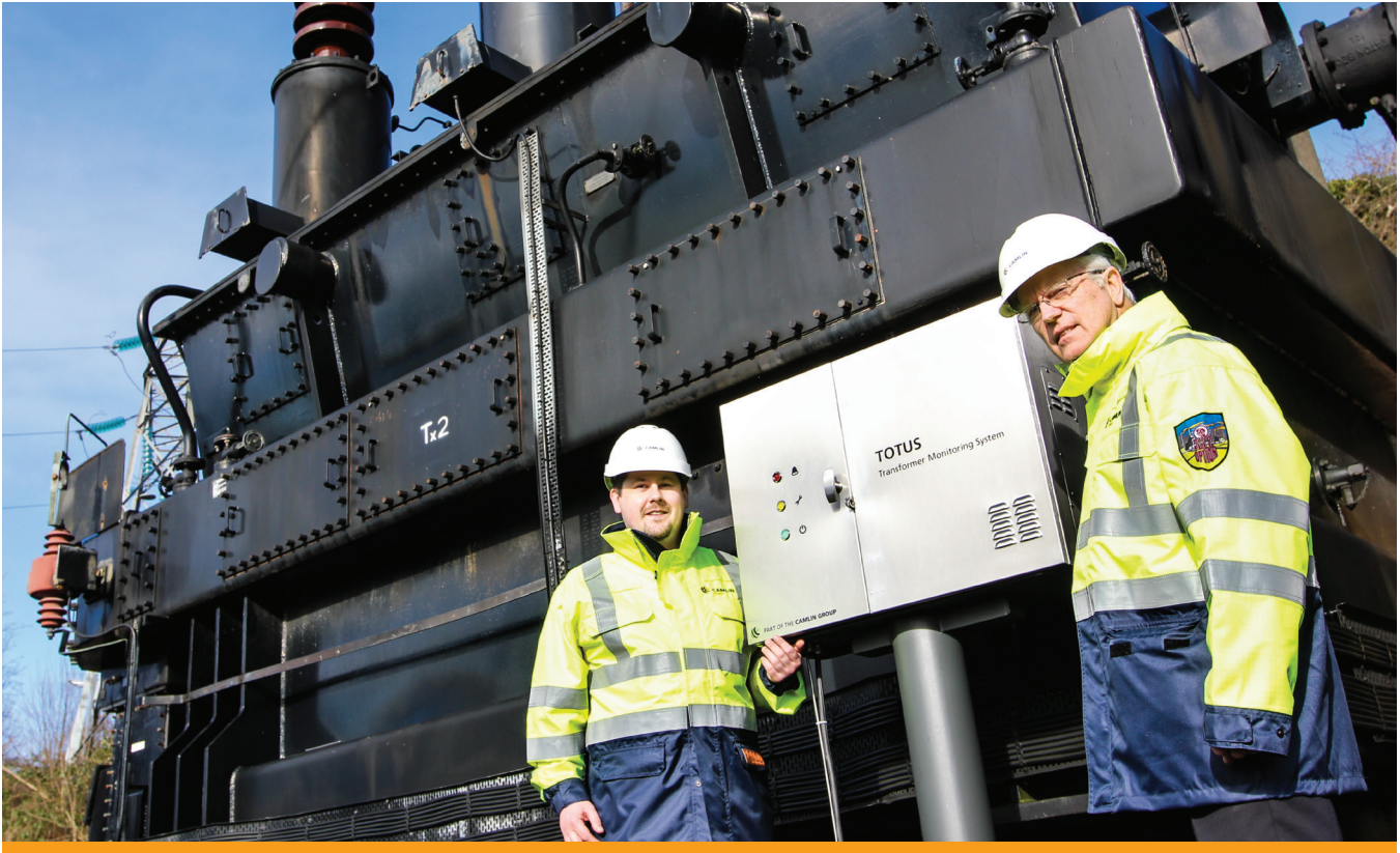
TOTUS DGA installed on a 110kV / 33kV transformer
