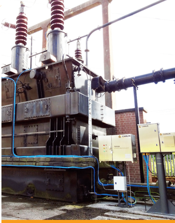
Camlin Power SIGMA TX installed on a 110kV / 33kV transformer
